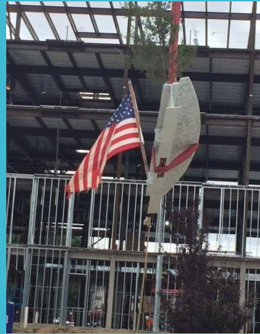
Left – "Topping Out" of the new Hospital construction June 20, 2018
